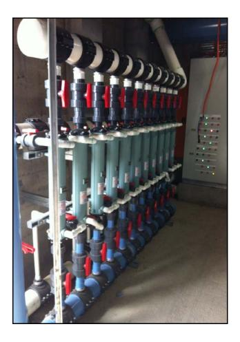
The Program and children's pools are on one filtration circuit which gets preferential heat from the residual artesian water. The set point for this plant is 31°C. Any useful heat remaining is then passed through the second bank of eleven heat exchangers which serve the 50 metre FINA pool. The upper set point for this plant is 28°C. Thermostats control heating boost pumps for both plants.
